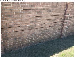
The following H columns need various degrees of mortar cracks repaired and some have loose stone that needs to be reset.
