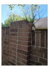
4 monument signs along Rapp Road: mortar cracks and missing mortar need to be repaired.
